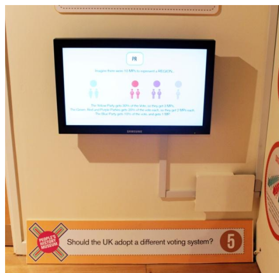
Figure 7 - An example of good wiring, with plug sockets covered and trunking keeping cabling neat.
